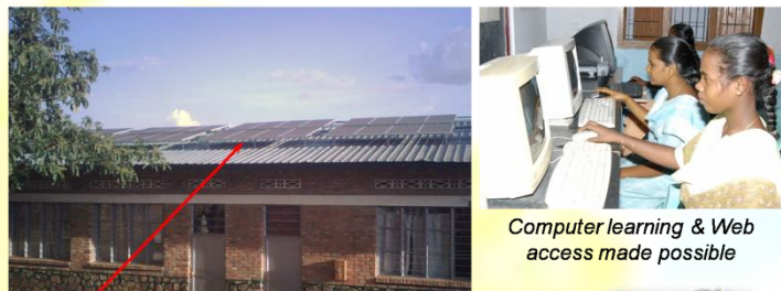
Roof-mounted Solar Panels
